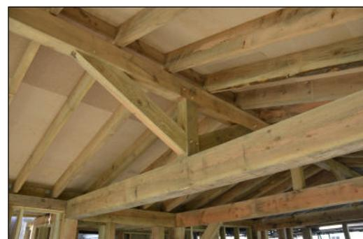
It's great to see the timber we cut from our own estate now being shaped, jointed, and fitted together. Here we have the main walls from the outside, and the rafters and ridge timbers from the inside of the building.
